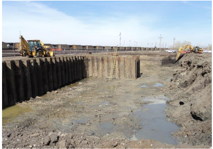
Excavation using sheet piling to protect active rail line in background.
