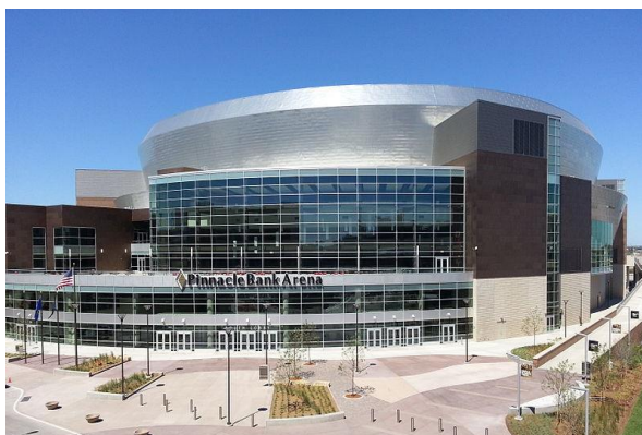
Pinnacle Bank Arena, September 2013
