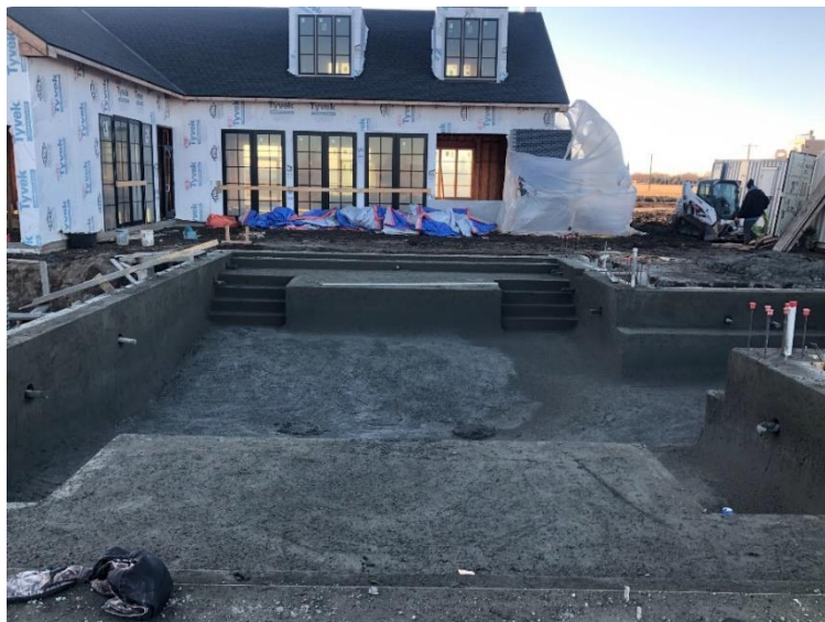
Swimming Pool Under Construction
