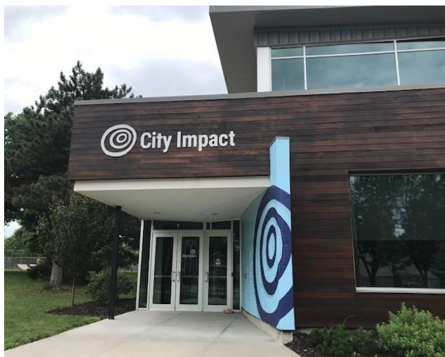
City Impact, a Lincoln-based non-profit, had all new LED lighting installed in 2021 with help from a low-interest loan through the DESL program.
