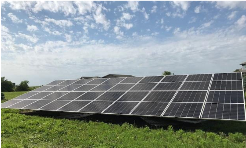
$35K Photo Voltaic Installation peaking 16,000 watts at 4 Seasons Farms, LLC in Ashland (June 2022).
