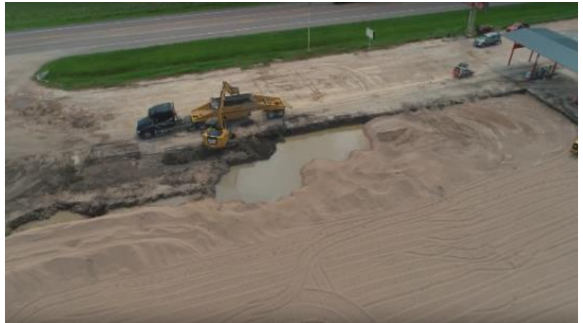
Large orphan site excavation in Minatare
