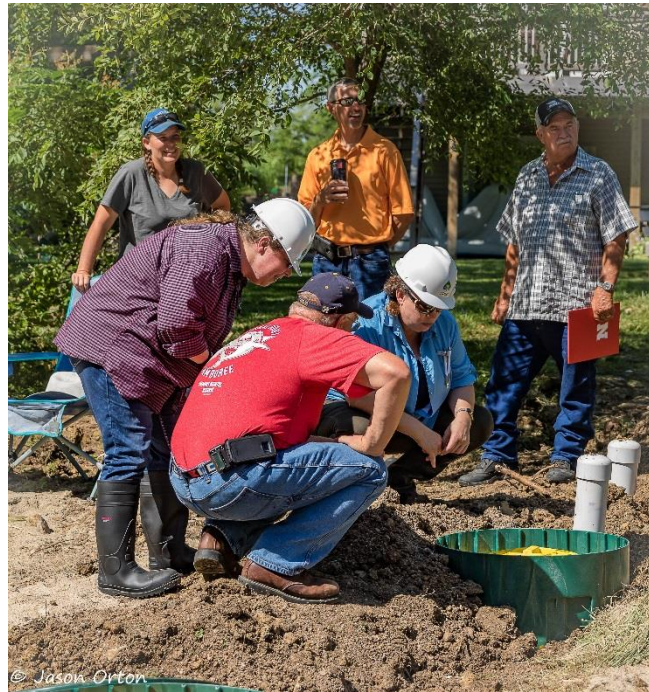
NDEQ Staff at a Mound System Installation Workshop
