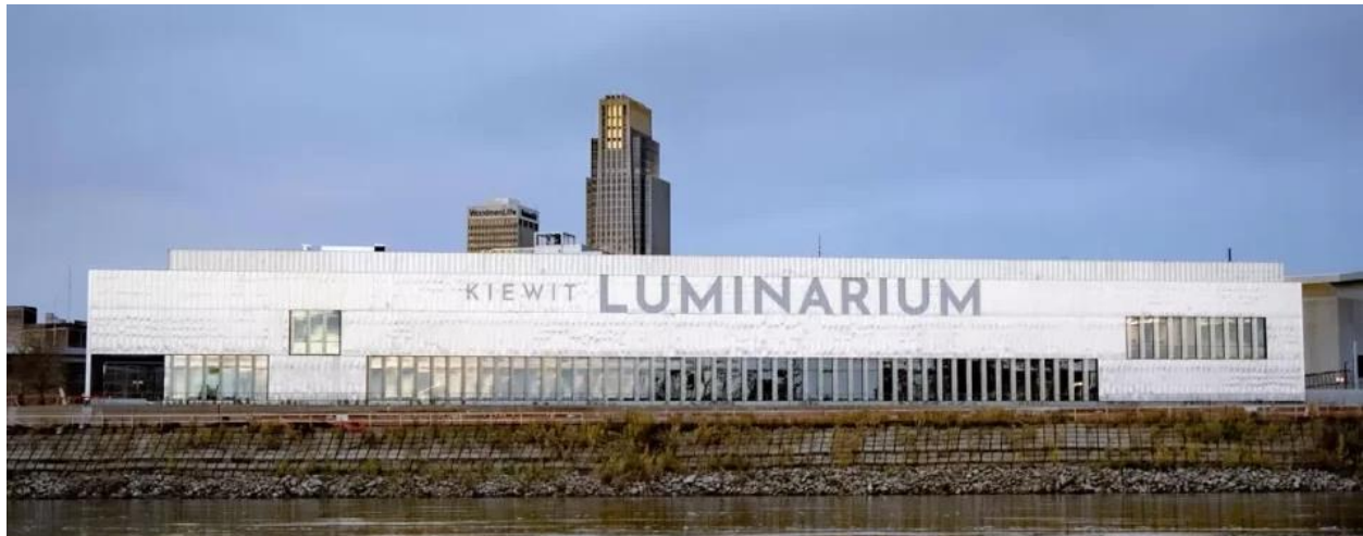
The photos on the top row show cleanup activities at the Lewis and Clark Landing Kiewit Discovery Center Foundation in Omaha. Remedial measures were taken during construction of the foundation of the Kiewit Luminarium to address and repair disturbances to the multi-layered protective capping system that was installed during cleanup of the American Smelting and Refining Company site (photos courtesy of the Remedial Action Report dated October 20, 2021). The photo on the bottom row shows the completed Kiewit Luminarium, which opened to the public on April 15, 2023, as a community space and interactive learning environment (photo modified from the Kiewit Luminarium webpage).
