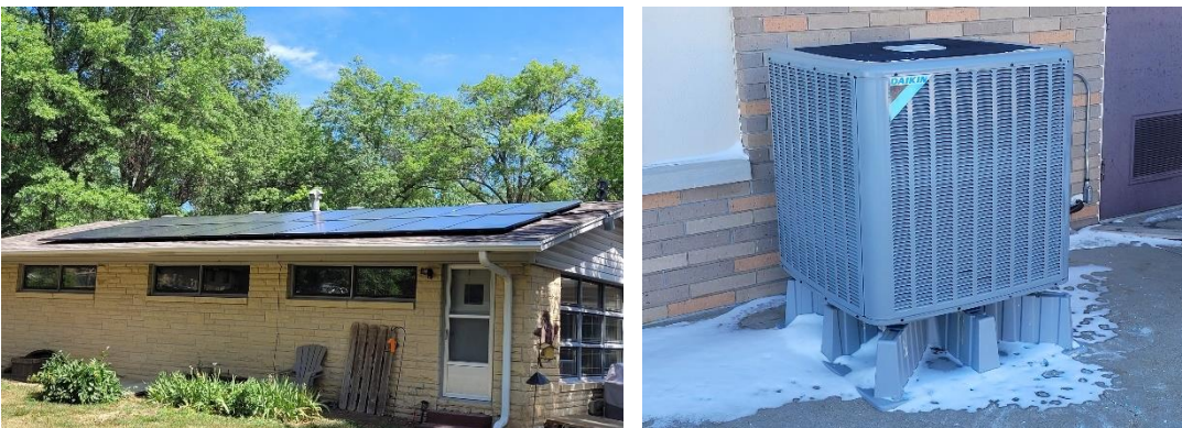
Left: A 7.2 kW Residential Photovoltaic system, Lincoln (2022); Right: A 5 ton, 16 SEER AC unit, part of a $320K HVAC project for Broken Bow United Methodist Church, Broken Bow (2022).
