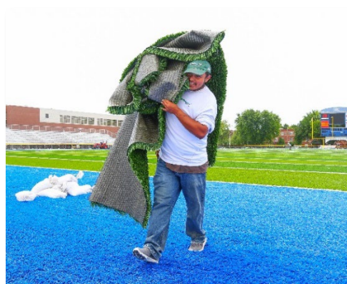
Photos provided by the University of Nebraska-Kearney. Artificial turf was installed on Foster Field in Cope Stadium. Crumb rubber from their old turf was reused. They saved $75,598 by reusing crumb rubber.
