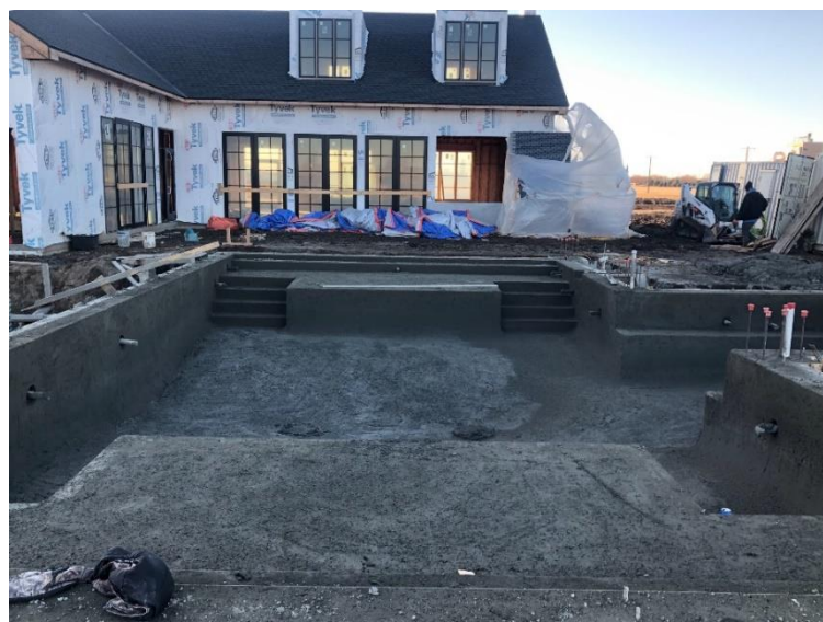
Swimming Pool Under Construction
