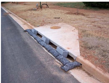
Typical rock bag inlet protection installation. Photo credit: Barry Tanning, Tetra Tech
