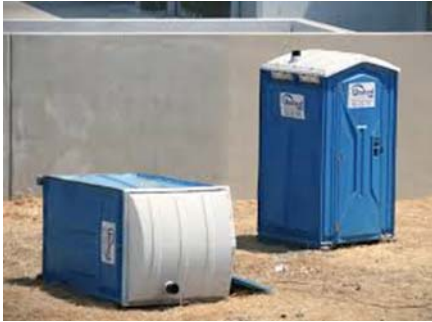
Position portable toilets so that they are secure and will not be tipped or knocked over. Photo credit: Kentucky Best Management Practices for Construction Activities, 2005
