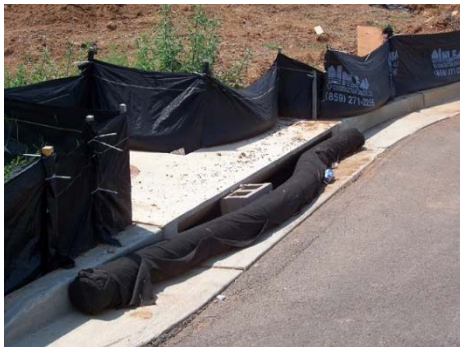
Typical filter bag inlet protection installation. Photo credit: Barry Tanning, Tetra Tech
