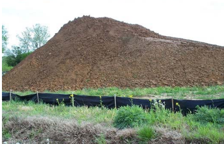
Silt fence around soil stockpile. Photo credit: Barry Tanning, Tetra Tech
