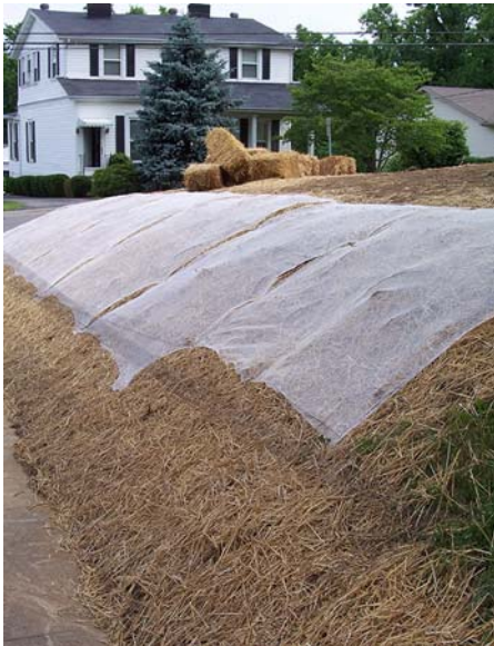
Example of adequate mulch coverage on 1sq.ft area. Photo credit: Maine DOT.
