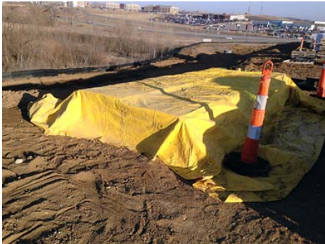
Cover materials using tarps or plastic sheeting to prevent precipitation from contacting construction site materials. Direct work crews to replace material stockpile covers at the end of the day and before rain. Photo credit: Barry Tanning, Tetra Tech
