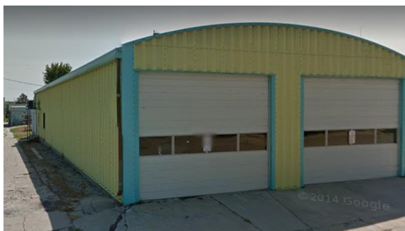
NDEQ used Section 128(a) Brownfields funding to complete a Phase I and Phase II Environmental Site Assessment and an Asbestos-containing Materials (ACM) Survey at the former fire hall building in the Village of Walthill. After the assessments were completed, additional funding was used to assist the village in properly removing and disposing of all ACM identified in the building. Having all of the environmental hurdles and uncertainties resolved allowed the small village to move forward and raise money for their new public library project.
