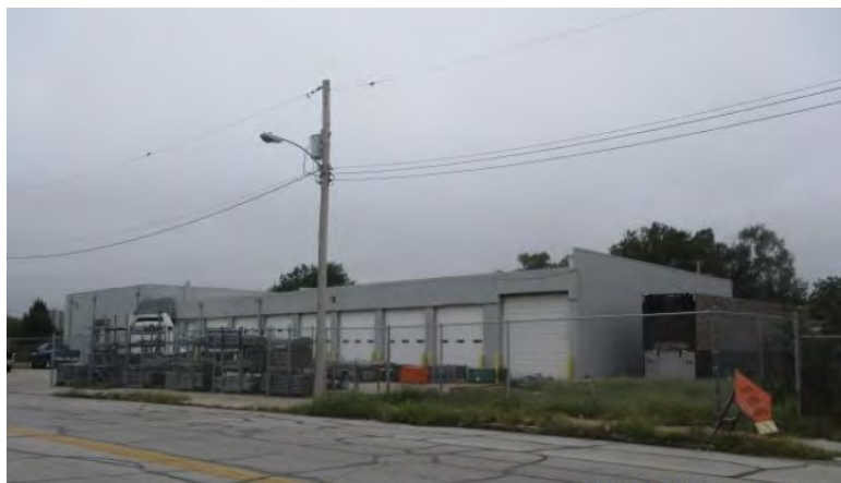
This former manufacturing facility located at 1528 N 16 th Street in Omaha will be the future location of a Tiny Houses project by Arch Icon Development and the Sienna Francis House. The City of Omaha enrolled the site in the VCP to address heavy metals contamination in the soil. When complete, approximately 50 tiny houses – each about the size of a hotel room – will be constructed onsite to provide a housing service for the homeless.
