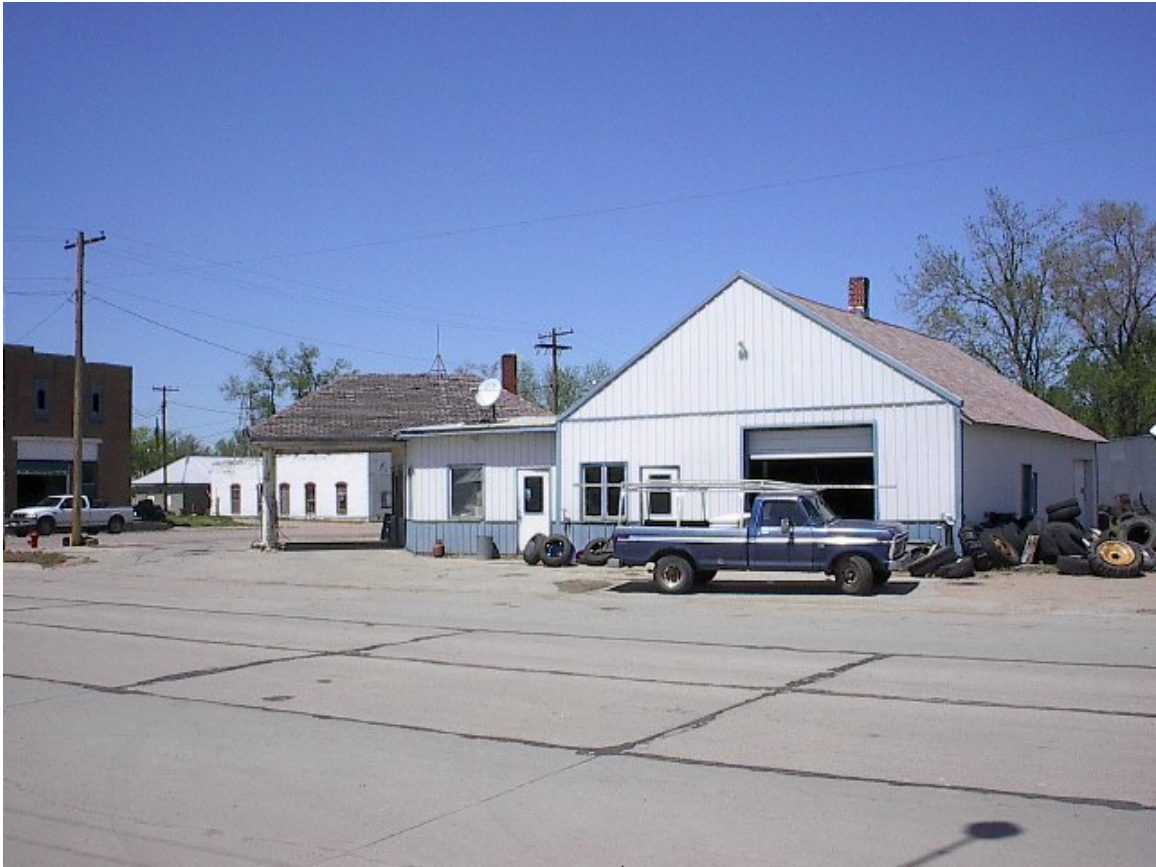
View of the south side of the D&H Property facing 1 st Street. Active product dispensers are present beneath the canopy.
